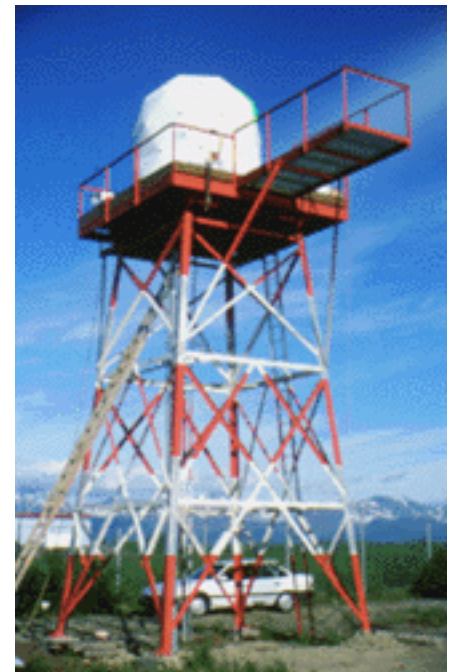
TRAD 8' Radome for HRPT download enclosure at the Anchorage International Airport. (Courtesy NWS Anchorage)
